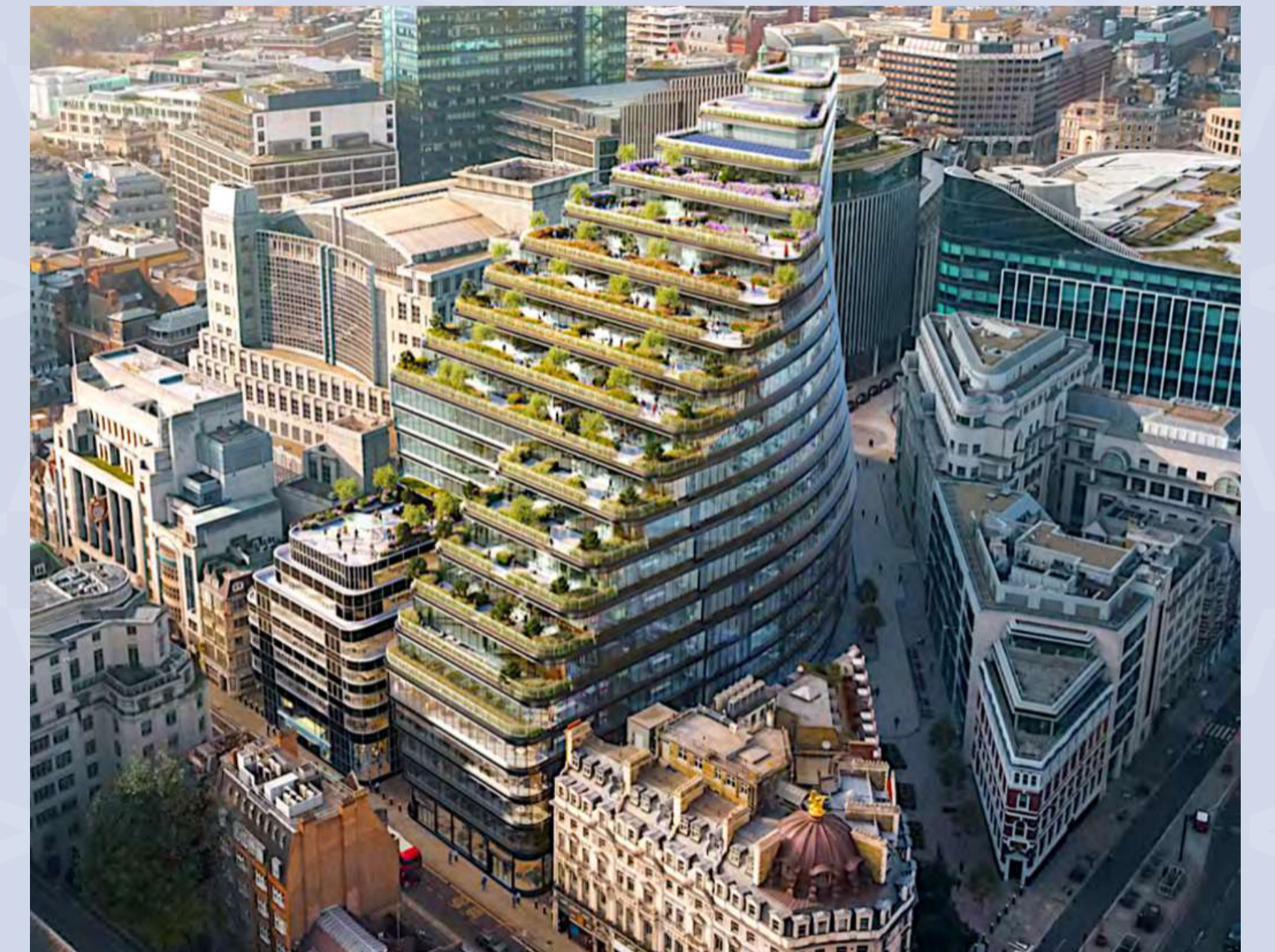
120 Fleet Street redevelopment
