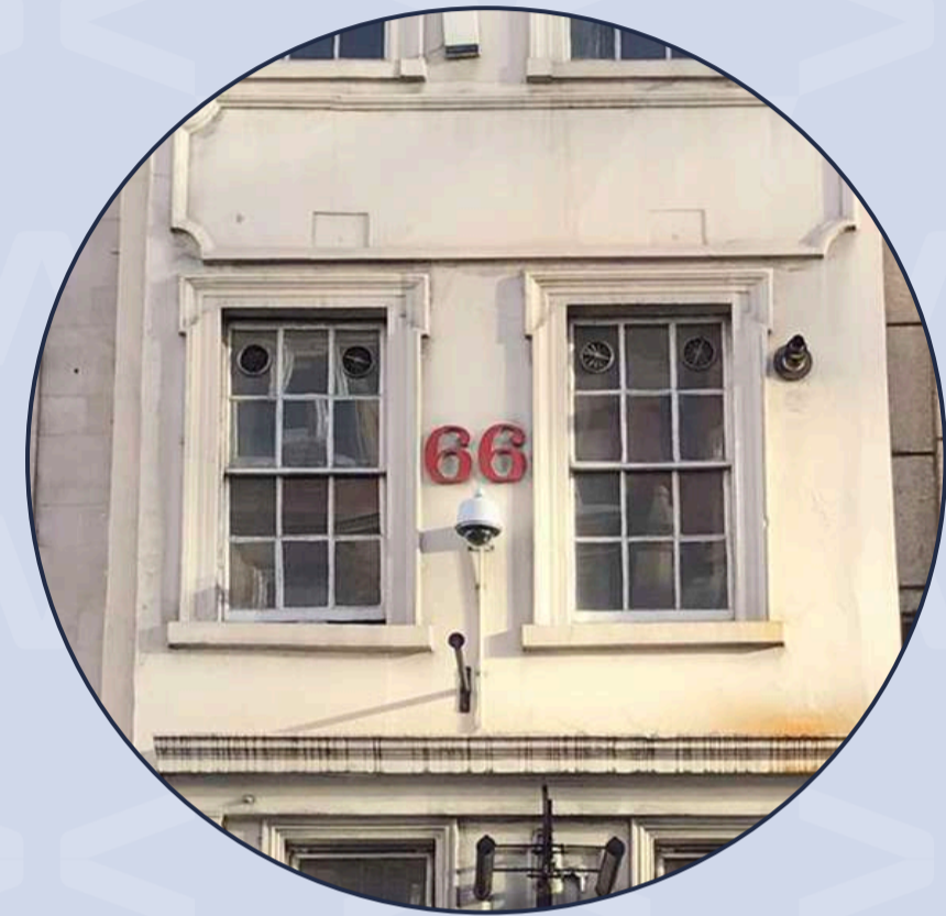
Repaired facade and windows to be made good
