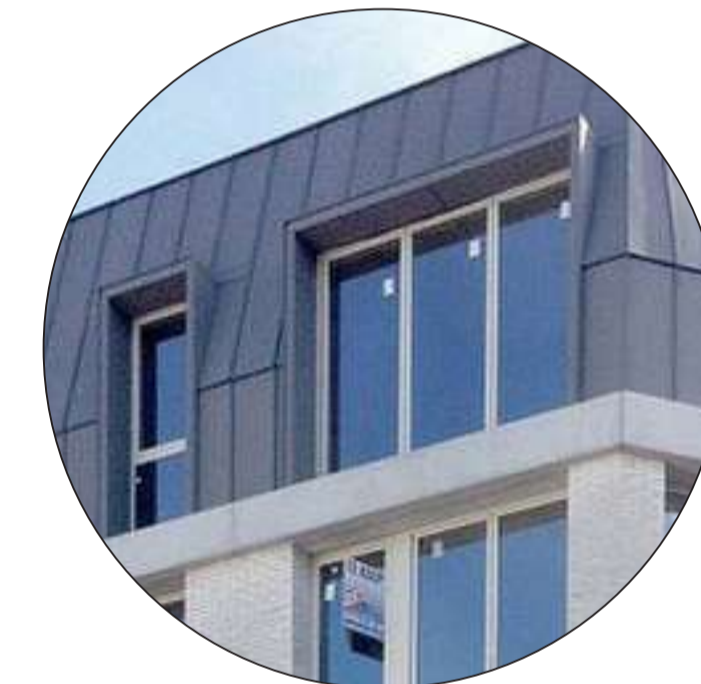
3. DORMER WINDOWS WITH STANDING SEAM MANSARD ROOF
